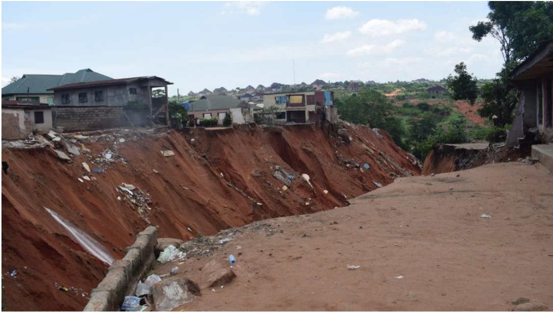
Figure 5. Erosion sweeps building in Agulu, Anambra State, Nigeria. Photo Credit: Linus Unah.
